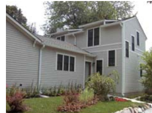
On this addition, a connection that is setback from the original structure, delineates the separation of new and old.
