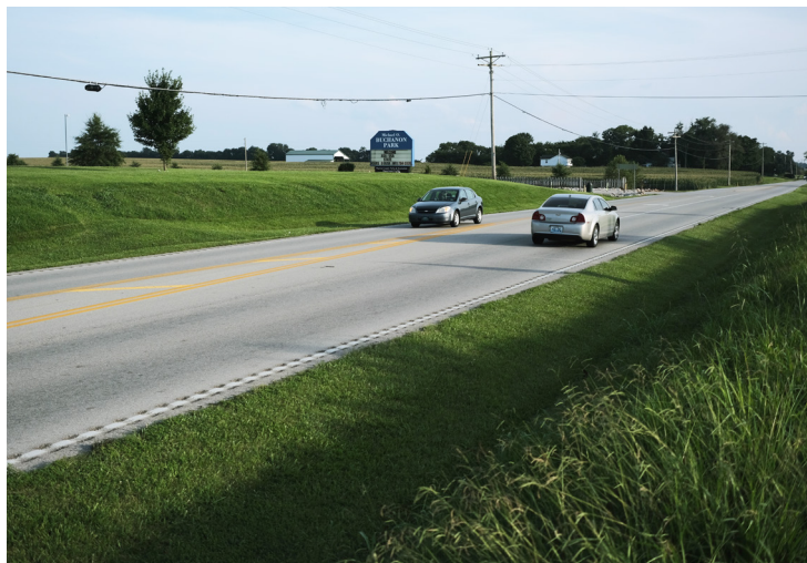
US 31W (Nashville Road), near Buchanan Park, traveling south toward Simpson County. KYTC is preparing for a widening project along this portion of roadway.
