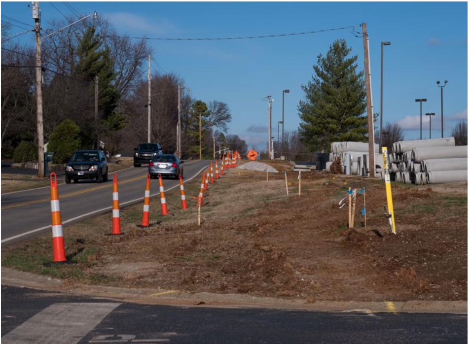
Construction gets underway on the Smallhouse Road widening project, Phase I, from Campbell Lane through the Highland Way intersection.
